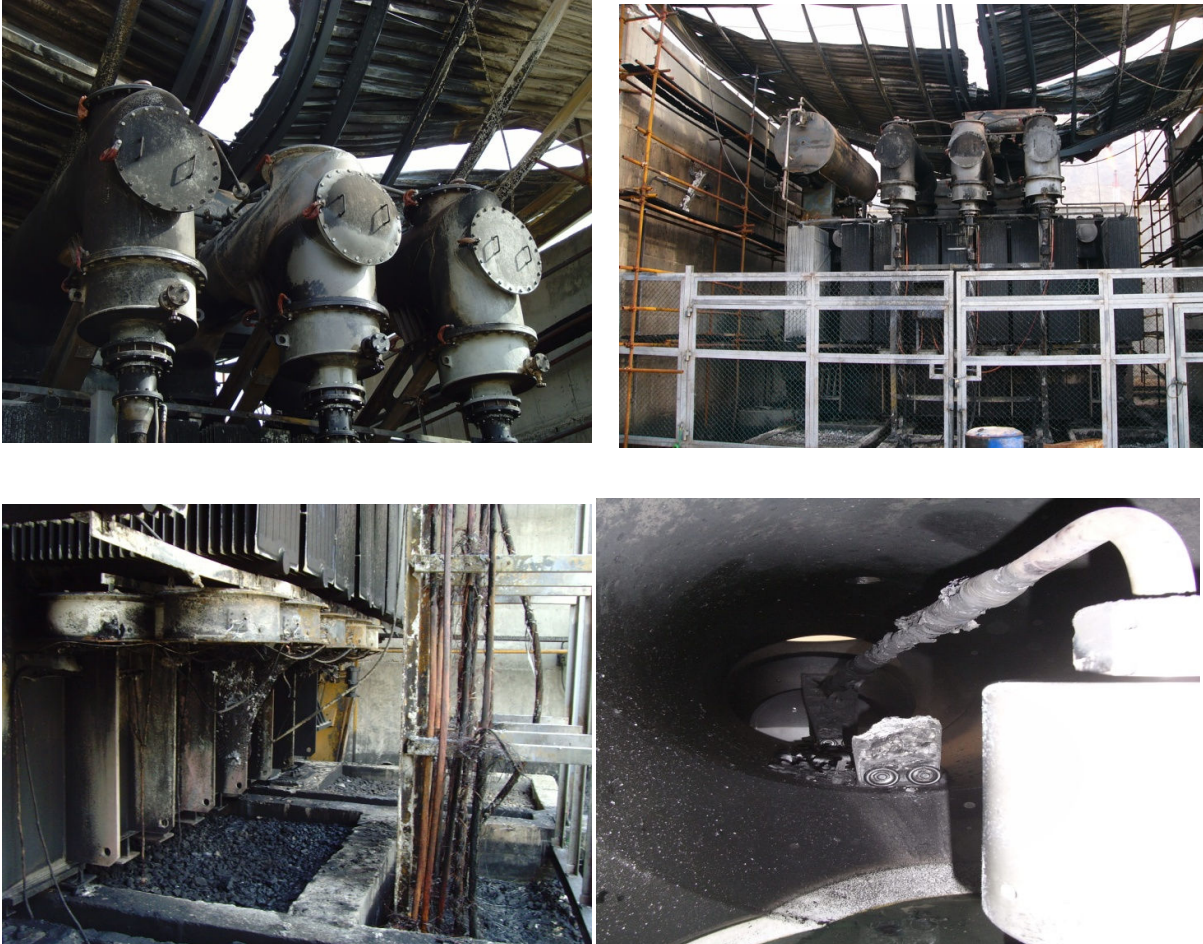
Figure 6: Transformer Damage
